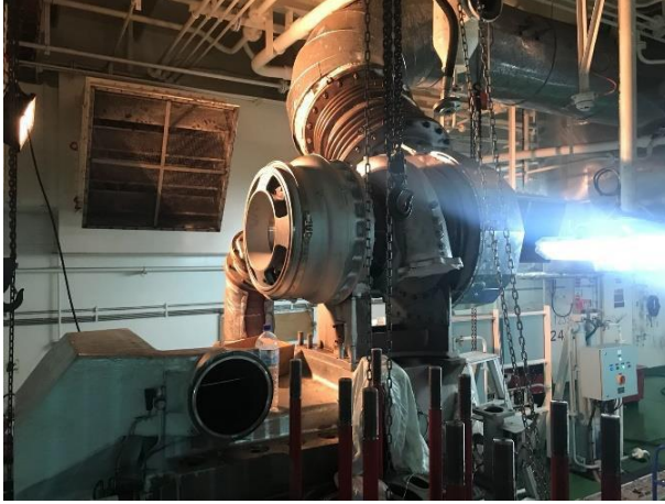
Damaged/New Turbocharger and Installation Works
