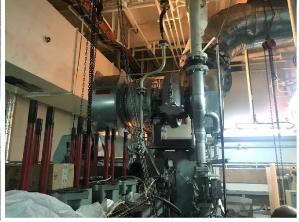
Damaged/New Turbocharger and Installation Works
